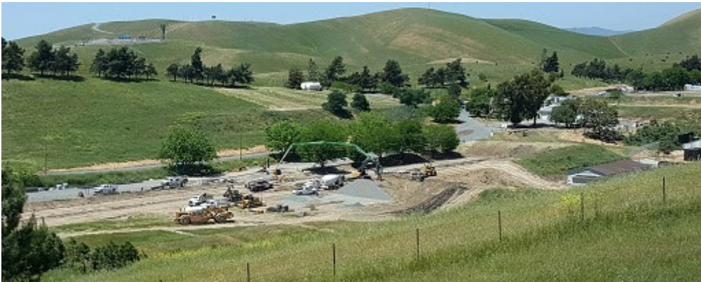
Range project view looking west from up the hill
